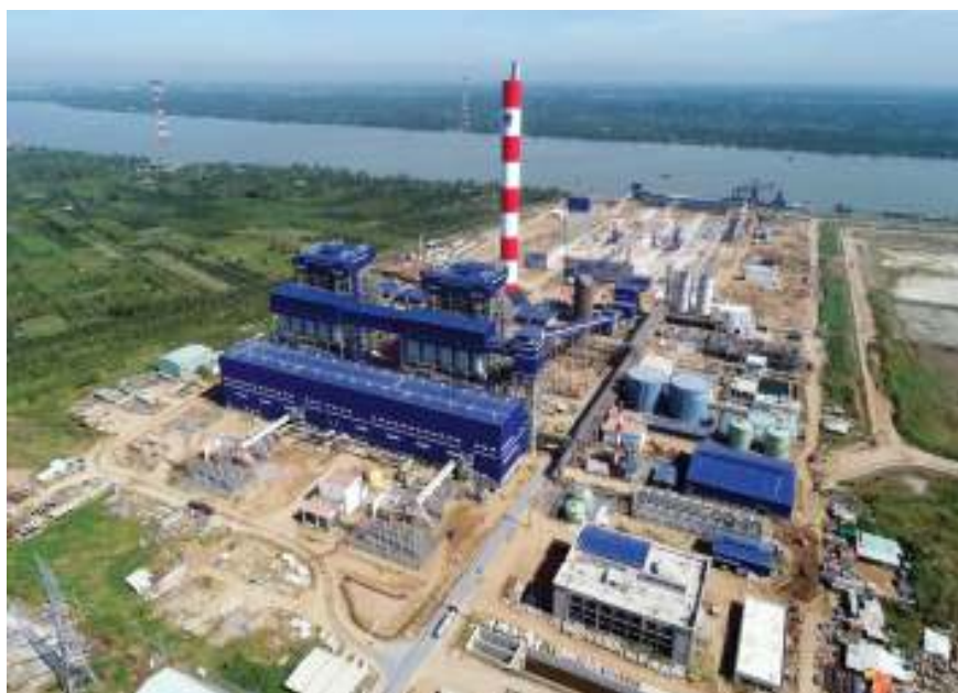
Song Hau 1 Thermal Power Plant Project is being gradually completed, and is expected to make great contribution to the local social economy
