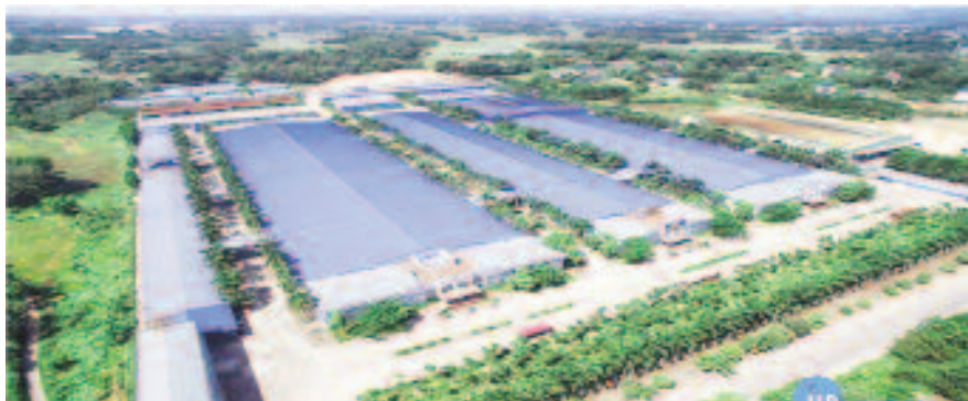
Co Chien Industrial Park, Vinh Long province
