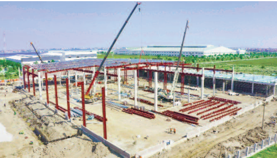
Deploying the construction of Toyo Plas Plastic Factory in Hoa Phu Industrial Park
