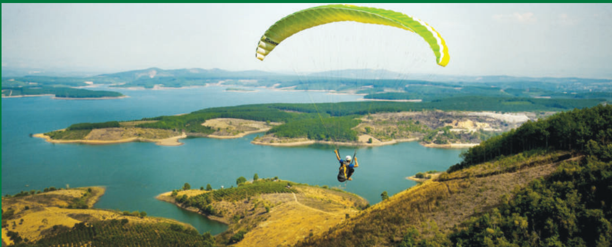
The reservoir of the Plei Krong hydropower plant
