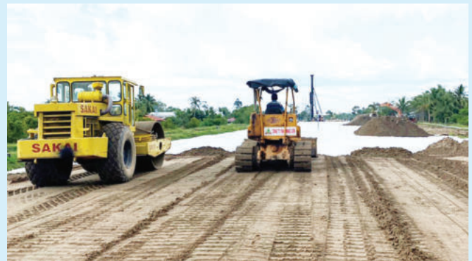
The rapid site clearance work for the My Thuan - Can Tho expressway project, the section through Binh Minh Town (phase 1) helps to ensure construction progress
