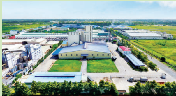
De Heus aqua feed factory - Vinh Long branch 1 in Hoa Phu Industrial Zone, Long Ho district - Vinh Long province
