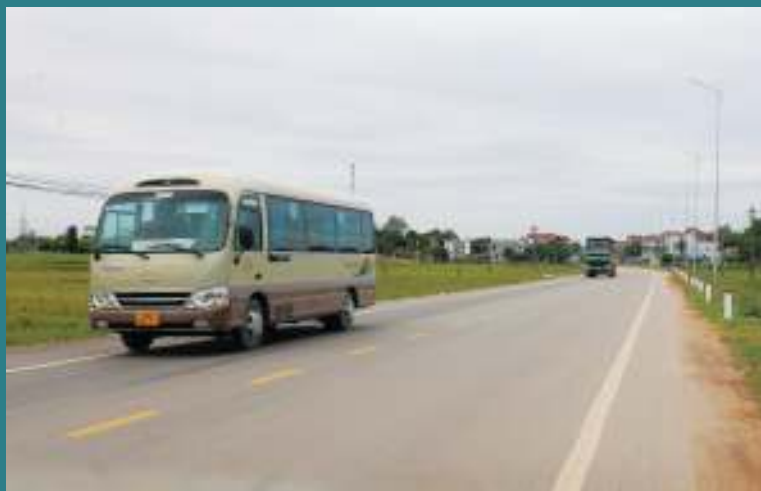
Project on the upgrading of National Highway 17, the section passing Viet Yen - Tan Yen districts
