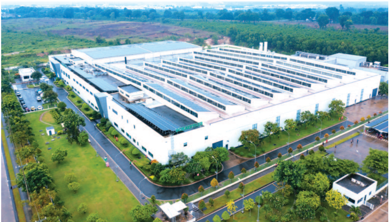
Solar power project at Schaeffler Vietnam's Dong Nai plant
