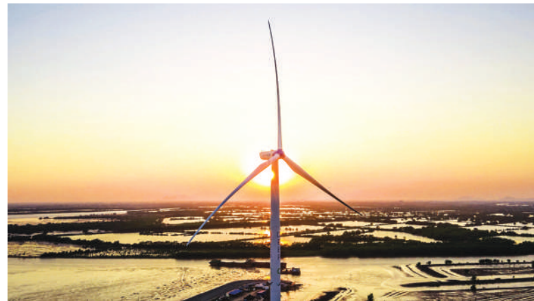
Wind turbine structure at the DEEP C Industrial Zone Cluster
