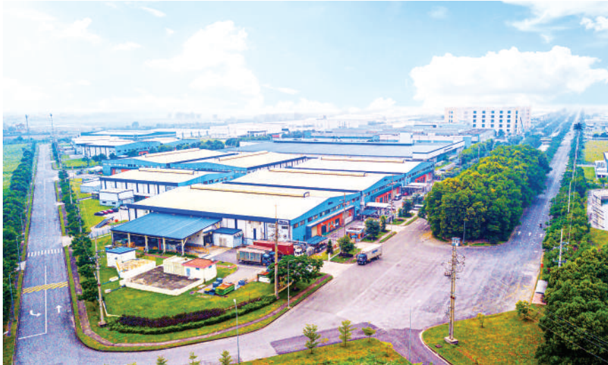
Bac Ninh Province is investing in logistics and infrastructure to strengthen its overall competitiveness
