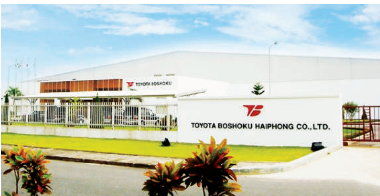
Renovation project of the Toyota Boshoku plant at Nomura Industrial Park, Hai Phong
