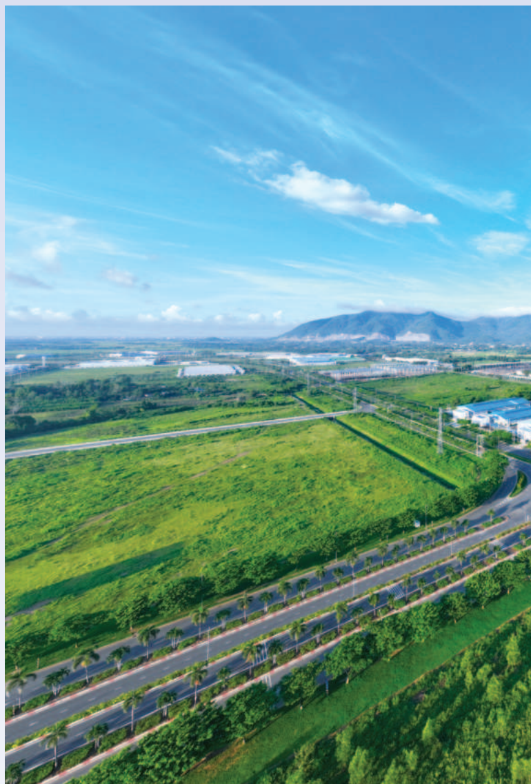
Sonadezi Long Thanh is actively utilizing its 51.6-ha industrial land at Chau Duc Industrial Park
