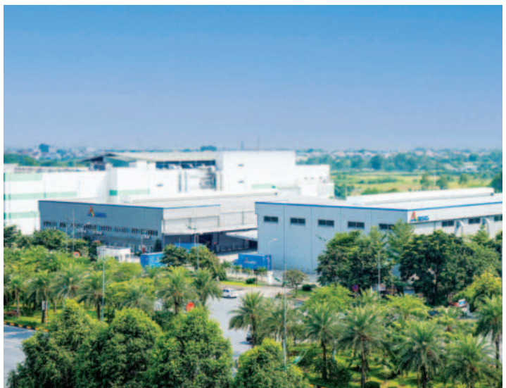
Headquarters of ASG Corporation at Logistics Services Center, Noi Bai Int'l Airport, Hanoi
