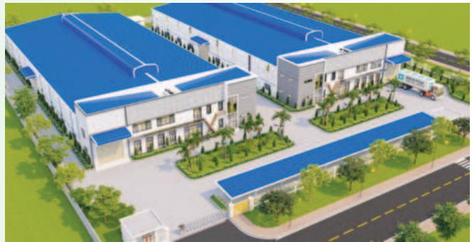
Sonadezi Long Binh's workshops meet high standards and are ready to serve diverse clients
