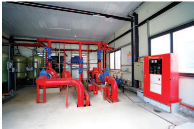
The company always puts quality and safety first
